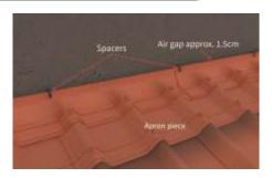
The ventilation gap between the wall and the apron piece should be secured with spacers that are applied at overlaps and in the middle of each apron piece.
